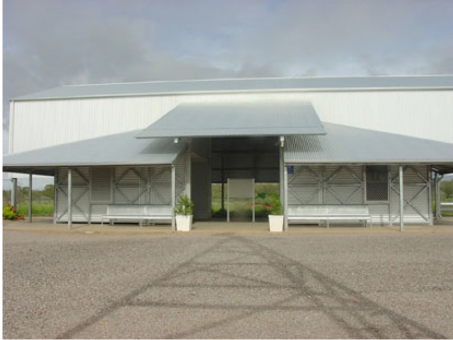
Replica of the original Croydon Railway Station built in steel in 2006 by Buchanan Architects
